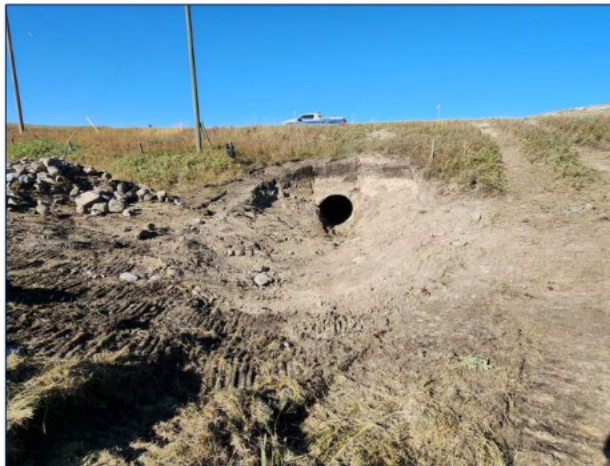
October 8, 2025 Upstream end with bevel section removed.
