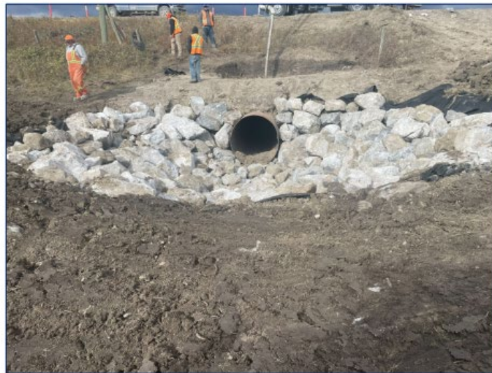
October 17, 2025 Upstream riprap installation completed.
