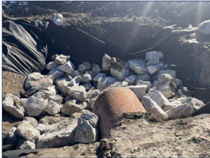
October 16, 2025 Upstream end clay seal backfilling completed. Riprap installation underway.
