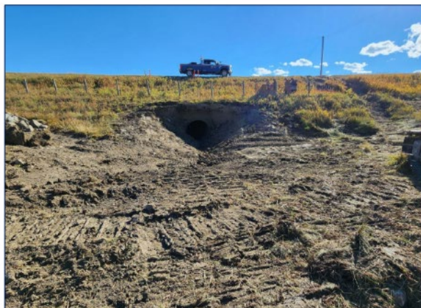
October 8, 2025 Downstream end with bevel section removed.
